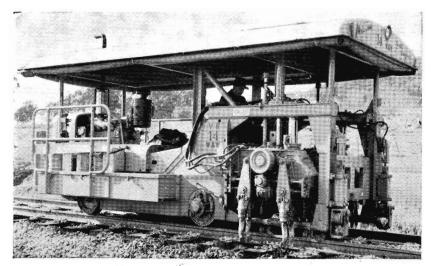
From Switzerland : This machine tamps ballast under the sleepers of the new standard gauge track at 1<sup>1</sup>/<sub>2</sub> miles a day.
