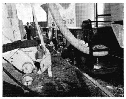
Hose connexions between rail wagon and road tanker. Air coming through hose at left blows flour into tanker through hose at right.
