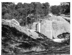
Sub-structure of a bridge over a valley at Belgrave to take the re-aligned broad gauge track to Belgrave. The bridge will be 60 ft. high and 225 ft. long.
