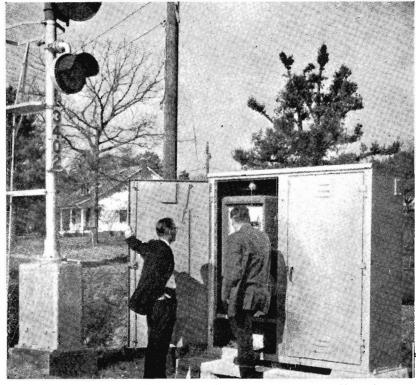
THE hotbox recorder-indicator panel being shown to a pressman. If a hotbox is detected, lower signal on mast automatically flags train.
