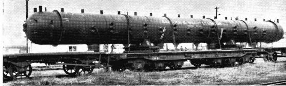
Equipment for S.E.C. power stations was carried over the Victorian Railways on Sunday, November 19. when the steam drum (*above*) and stator (*below*) were taken from Appleton Dock to Yallourn. The stator, an out-of-gauge load on the well wagon, weighs 116 tons and is 14' 9" high ; the 100-ton steam drum is 86 ft. long.
