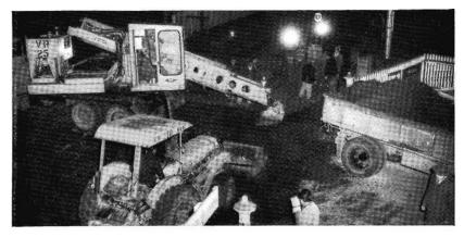
Gradall excavator cleans out ballast from road bed.
