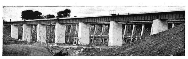
This impressive bridge over Mt. Emu Creek, between Boorcan and Terang, was recently completed by district Way and Works Branch staff. On a new alignment of track, it replaces the old (1887) timber bridge seen in the background. With eight 63-foot spans and three of 40 feet, it has a total length of 624 feet. All the piers are founded on concrete shell piles, some going down to 50 feet. The concrete structure will need much less maintenance than timber. (Photograph: Warnambool Standard).
