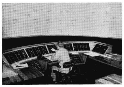
DISTRIBUTION of electric power on the Gippsland line is controlled from this Power Operation Room at the Warragul Electrical Depot. Warragul Electrical Depot . . a somewhat inadequate name, for it in no way signifies its importance. This modern partly air-conditioned two-storey building, in a setting of colourful homes and gardens, houses the Power Operation Room, the Supervisory Equipment Room and the Overhead Depot.
