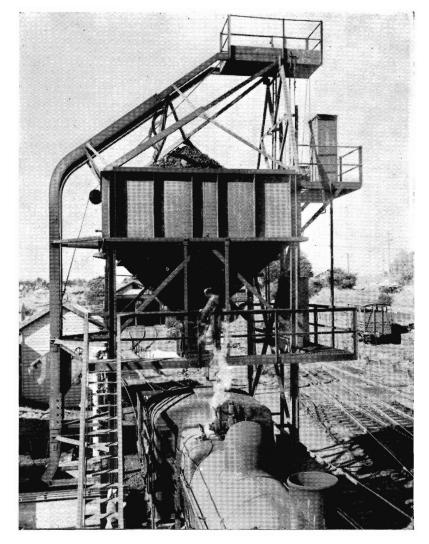
Korumburra loco. depot's automatic coal stage. State Mine coal falls from adjoining hopper wagons through a grille. It is then loaded into a 15 cwt. capacity bucket that then rises and empties—the three operations being automatic—into the 50 ton capacity hopper. From there the coal empties from the bottom of the hopper into the loco. tender, under manual control.
