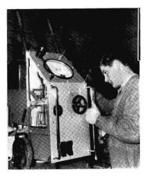
ANOTHER recent example of the skill of the Electrical Testing Division's staff: they designed and built this high voltage portable tester for checking electric equipment on suburban carriages. Apprentice Electrical Fitter P. Lawrence is engrossed in his work.
