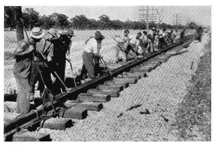
Standard gauge creeps nearer Melbourne. Close to Benalla this 90 ft welded rail is being turned into position after which it will be " pinned " down by the pre-driven dog-spikes. In the right of the picture can be seen the metalled edge of the existing 5ft. 3in. gauge track.
