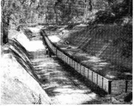
With the completion of the new, curving platform at Tecoma, foundations are being laid for the station buildings. Entrance to the station will be by means of a ramp.
