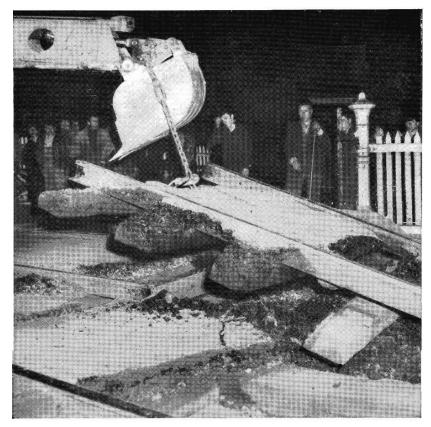
The Gradall excavator is used not only for excavating and filling, but also for lifting out sections of old track, as shown above, picking up and loading sleepers, etc.
