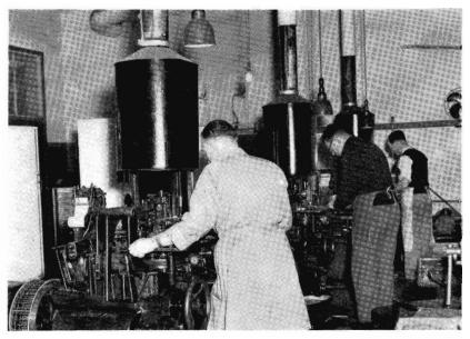
Casting type at the V.R. Printing Works
