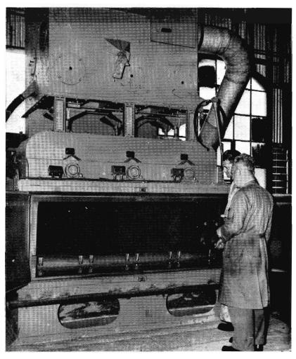
Shot peening machine with doors opened to show roller on which springs are placed.
