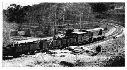
Sleepers being discharged at a point between Upper Ferntree Gully and Upwey. The former level crossing at this location has been replaced by overhead rail bridge.
