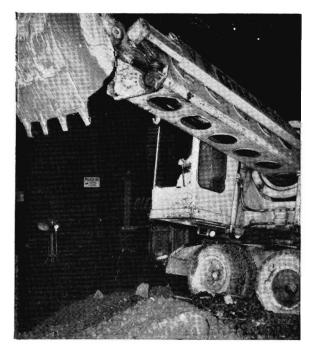
The steel jaws of the Gradall can lift over half a ton at one bite.
