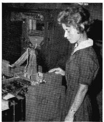
Powers-Samos "interpolator" interleaving or extracting punched cards from files for further processing by tabulators.
