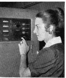
Electronic multiplying punch that senses information from punched cards, makes mathematical calculations and punches answer into the card.
