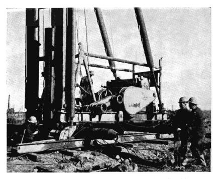
Standard gauge progress : pile driving at South Kensington for rail weighbridge in forwarding agents' area. Some of the piles have been driven to a depth of over\_90 feet.
