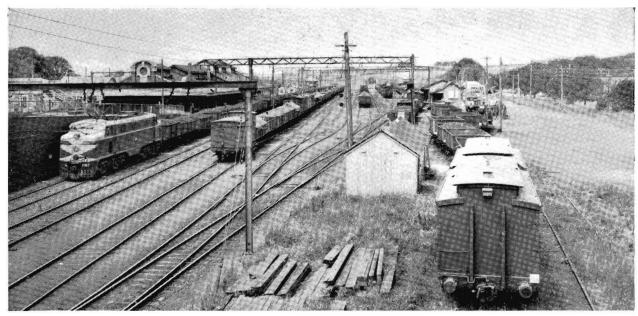
WARRAGUL, of which this is a general view of the goods yard, was the terminal point of the V.R.'s first country electric train service introduced in 1954, and since extended to Traralgon. A long brown coal and briquette train, hauled by an L class electric locomotive, is just leaving for Melbourne.
