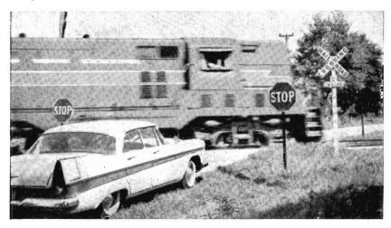
A 75% reduction has been made in the annual number of accidents at 313 railroad crossings of secondary highways in the State of Michigan, U.S.A., by installing red and white octagonal "stop" signs (above) at crossings protected only with the conventional crossbuck signs.
