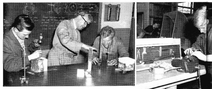
(Above) Apprentice Fitters and Turners N. Parfitt and J. Stevenson being taught by Instructor J. Mitchell in the marking out of a chipping block exercise. (Right) Performing the finishing operation on a "G" clamp is Apprentice Fitter and Turner P. Browning.
