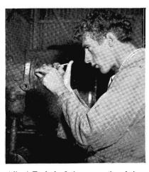
(Above) Typical of the apprentices being given practical training at Bendigo North Workshops, Apprentice Fitter and Turner R. Lawrence concentrates on the precision maintenance of a brake triple valve.
