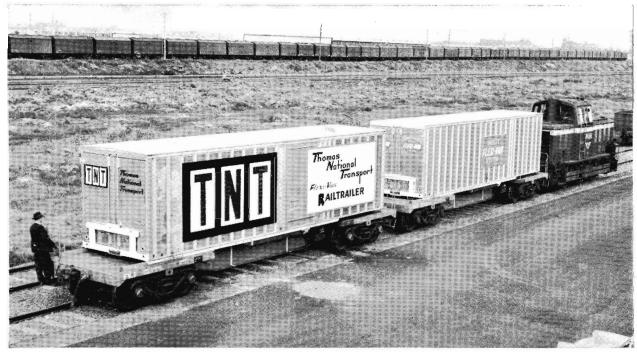
Flexi-vans being hauled by W class diesel-hydraulic locomotive for marshalling on daily Adelaide fast freight train.
